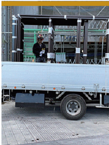
Figure 1.3.1.1-7 Reading RFID tags when receiving construction components
