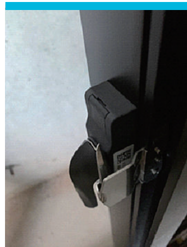
Figure 1.3.1.2-2 RFID tag attached to the frame of a window
