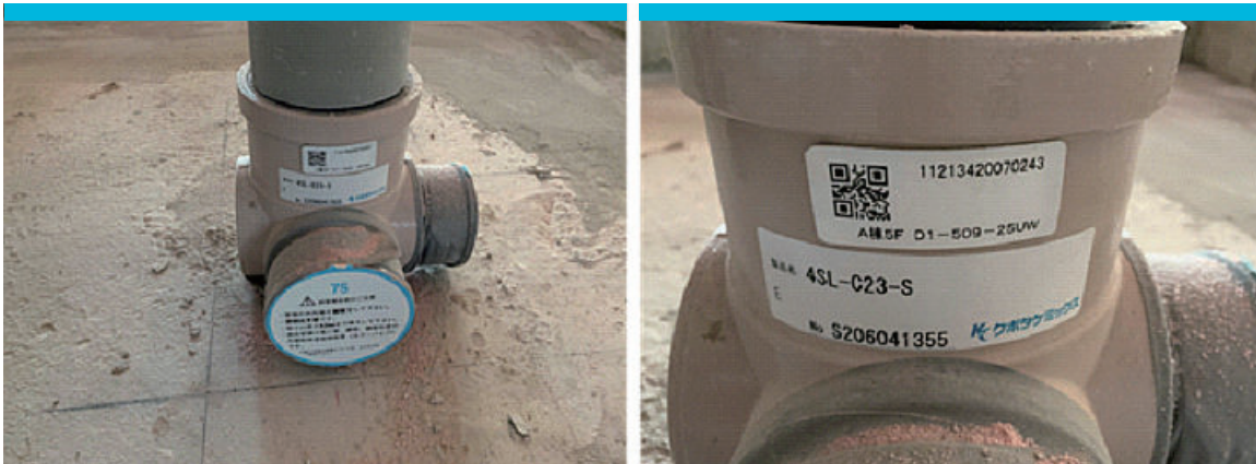
Figure 1.3.1.1-1 RFID tag attached to a connector for drainage pipes
