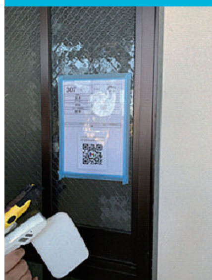
Figure 1.3.1.1-2 QR code for location information at a room entrance
