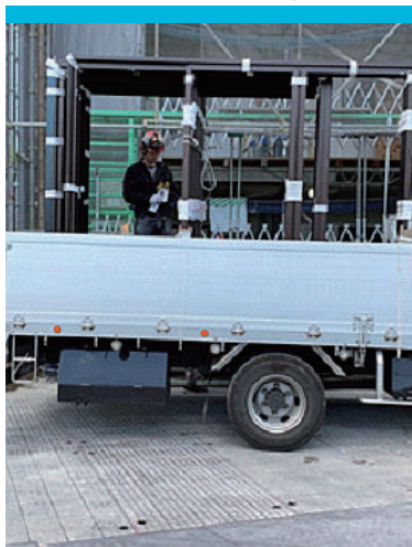
Figure 1.3.1.2-4 RFID reading at the reception of construction components
