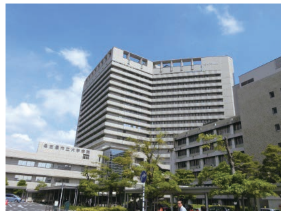
Fig. 1.2.1-1 Nagoya City University Hospital
